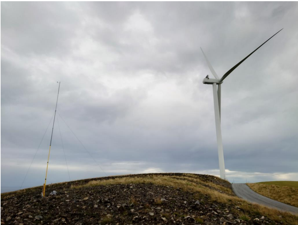
Figure 1-3: Wind turbine T07 and the 10 m tall weather mast
